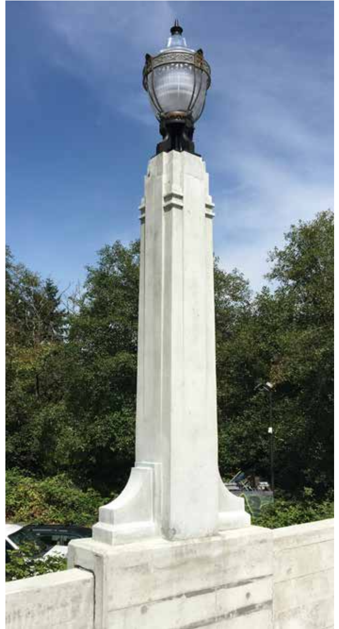
Replicated lamp standards from the original 1932 designs (removed in the 1960s), all-new art deco concrete standards with bronze light fixtures – copied from an original surviving fixture example – now restored into their 74 original positions along the bridge. Photos Heritage Vancouver Society
