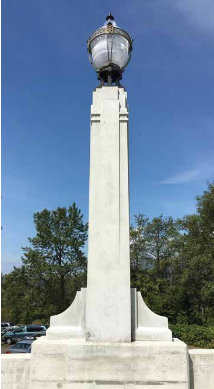
Replicated lamp standards from the original 1932 designs (removed in the 1960s), all-new art deco concrete standards with bronze light fixtures – copied from an original surviving fixture example – now restored into their 74 original positions along the bridge. Photos Heritage Vancouver Society
