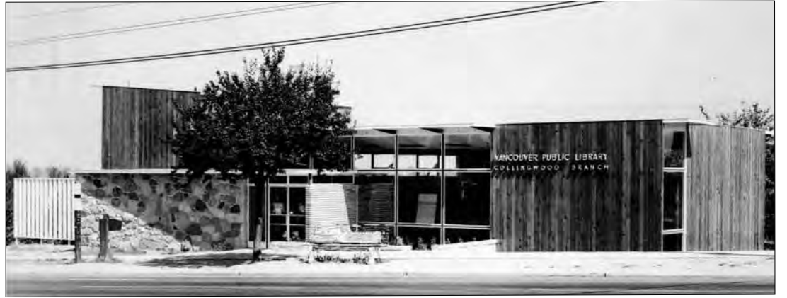
An extraordinary photo of Vancouver Public Library's Collingwood branch as it appeared before its opening in early July 1951. The glass expanse at the front of the building has since been covered up in a subsequent renovation. (Source: Vancouver Public Library, Special Collections, VPL 8856)
